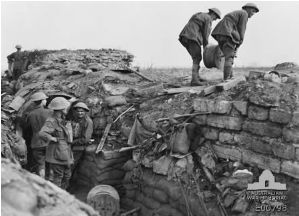
Above: Sappers laying telephone cable in the Menin Road, Belgium area, September 1917
