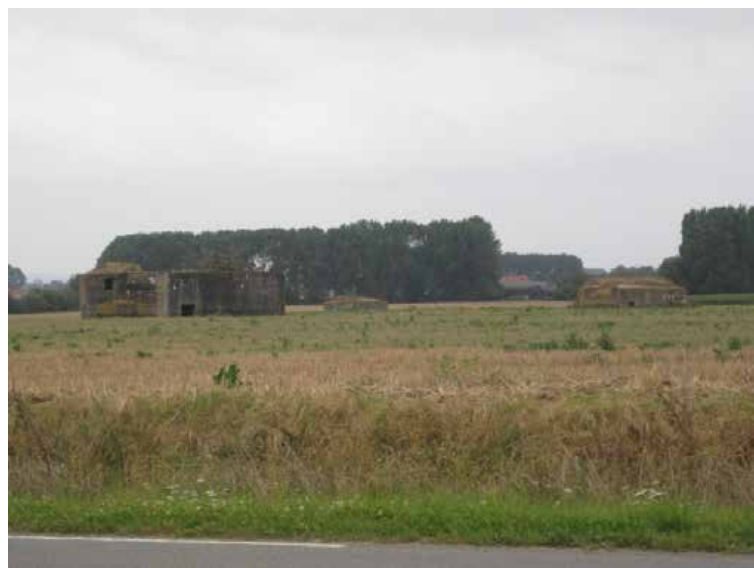
Abandoned blockhouses in a field near Fromelles, 9/2012.
