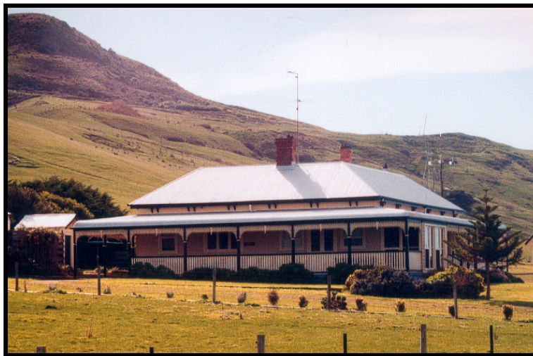
House at Browns Creek, Site #228
