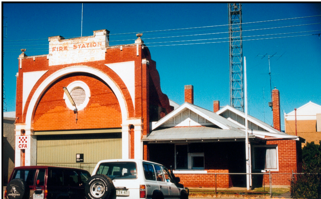
Fire Station & Residence, Colac Site #158
