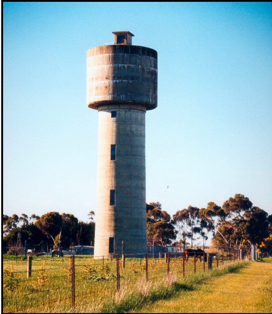
Cressy Water Tower Site #172
