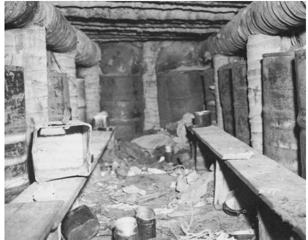
Inside of a typical Japanese bunker at Buna. The small space between the top of the drums and the log above them was ample for use as a firing slit
