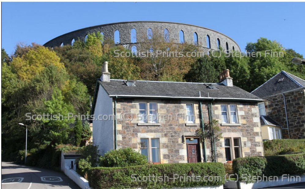
Amazingly, this exact view is still intact !
