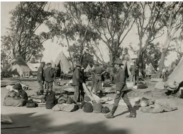
Blackboy Hill Camp - Trainee Soldiers erecting Tents AWM H16151
