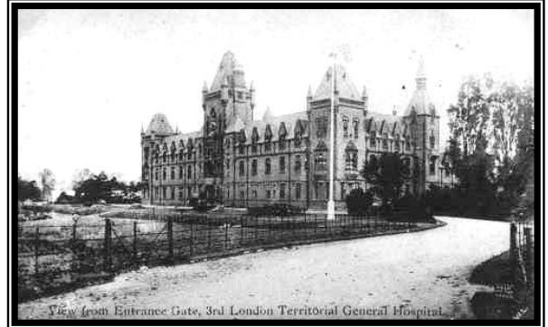
Figure 35: Above - Wandsworth Hospital, London
