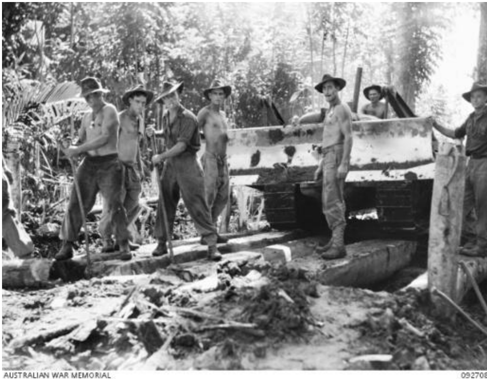
Figure 15: Wewak Area, New Guinea. 1945-05-30. Members of 2/2 Field Company Royal Engineers and 2/8 Infantry Battalion using a bulldozer to clear debris and mud during preparation to bridge a creek.
