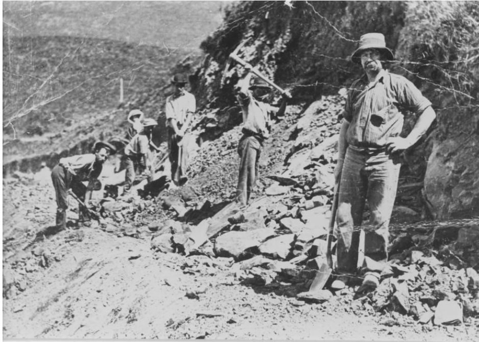
Men working on the construction of the Great Ocean Road
