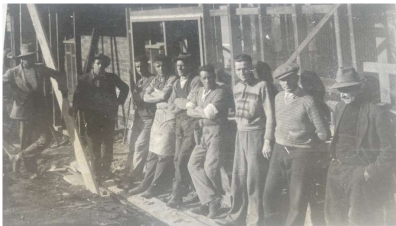
Building operations Lorne 1933. Harry rolled up sleeves.
