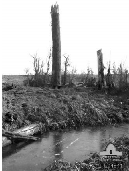
Observation post made of steel and disguised as a tree. Messines area, 1918. (AWM E 04541)
