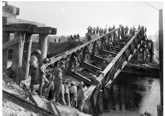
Fig 4. Possibly Oliver, whilst repairing Chipilly Bridge.
